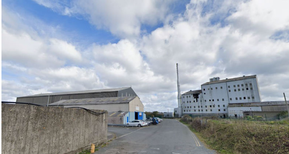
Fig No.5 View of existing building on site as viewed from the south.
